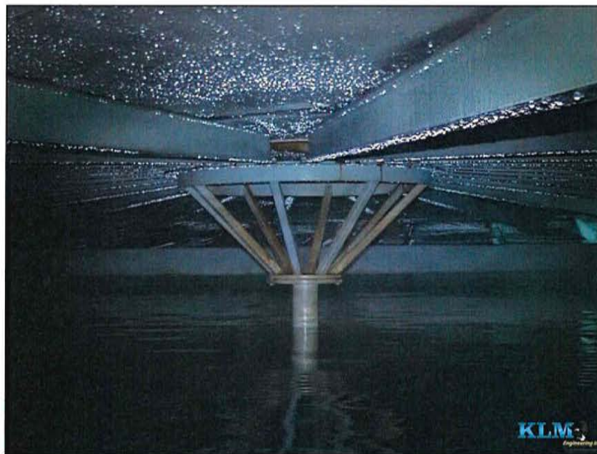
Photo No. 2 View of roof and center support column
