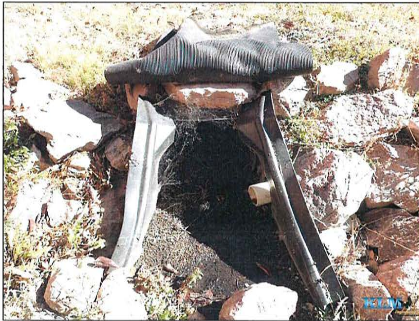
Photo No. 23 Overflow pipe outlet
