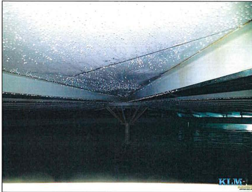
Photo No. 3 Condition of roof rafters and roof plates
