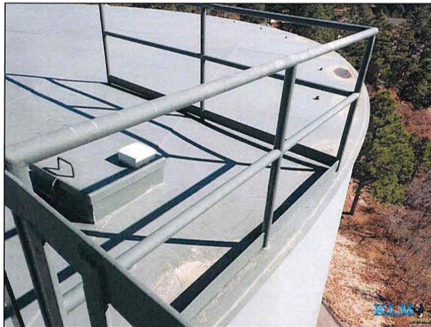
Photo No. 18 Condition of handrail
