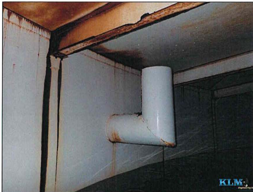
Photo No. 10 Condition of shell Overflow pipe visible
