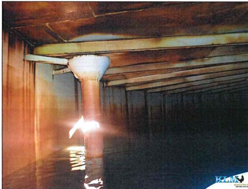
Photo No. 7 Condition of roof, overflow pipe, and shell
