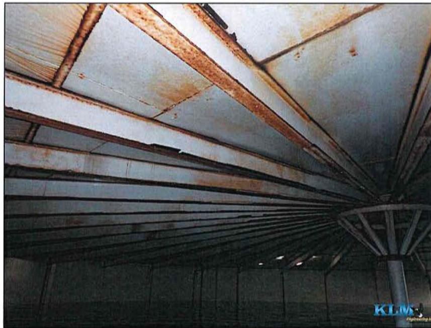
Photo No. 6 Condition of roof rafters and roof plates
