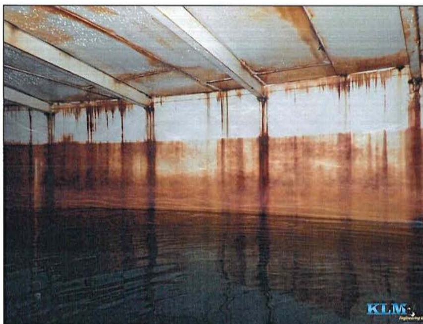
Photo No. 8 Condition of shell
