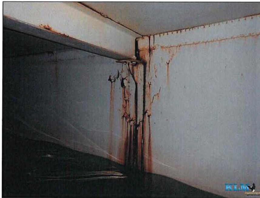
Photo No. 9 Condition of shell
