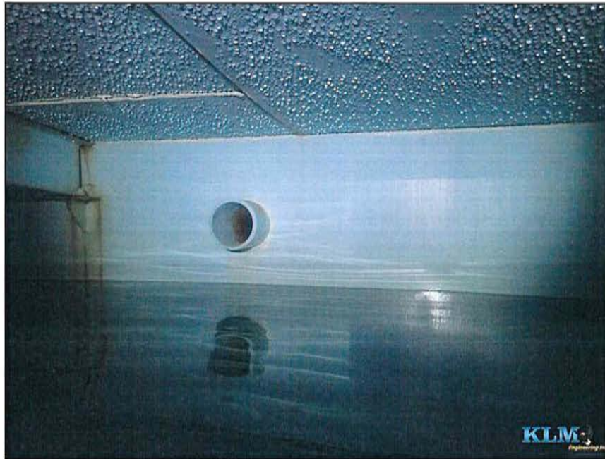
Photo No. 7 Condition of shell Overflow pipe visible
