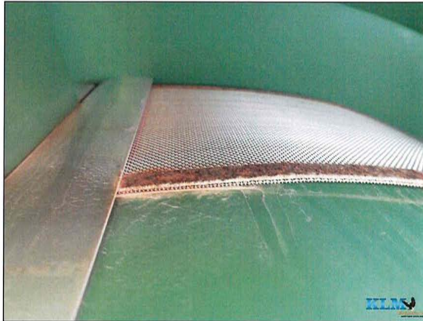
Photo No. 13 Condition of finial vent
