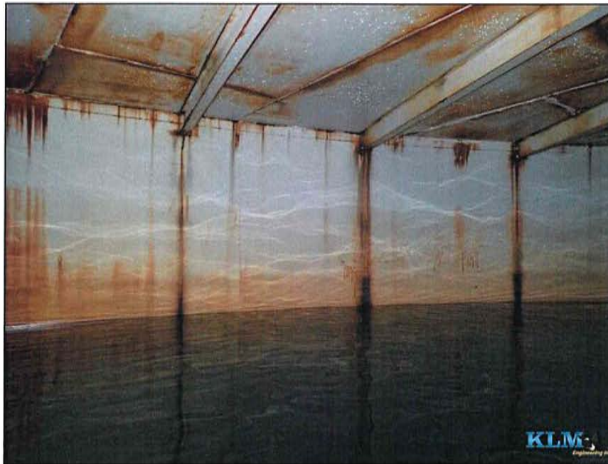
Photo No. 9 Condition of shell
