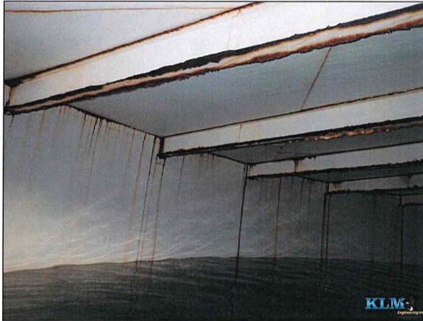
Photo No. 9 Condition of shell
