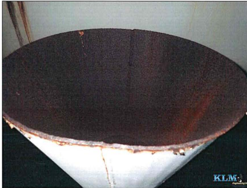
Photo No. 11 Condition of overflow pipe
