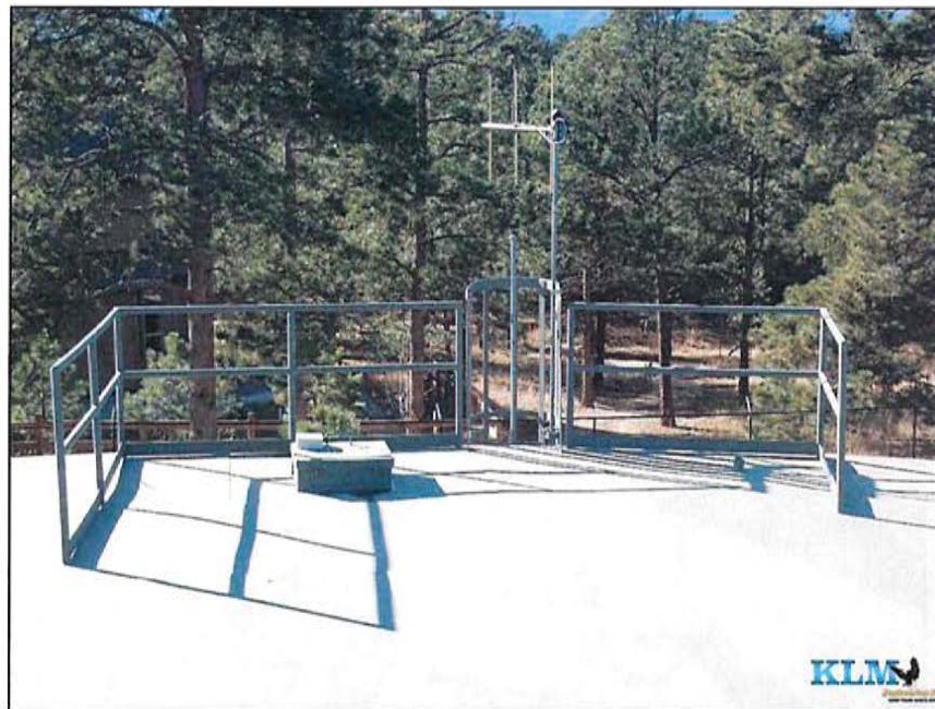
Photo No. 14 View of roof handrail and wet access manway
