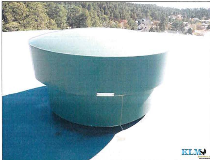
Photo No. 12 Finial vent
