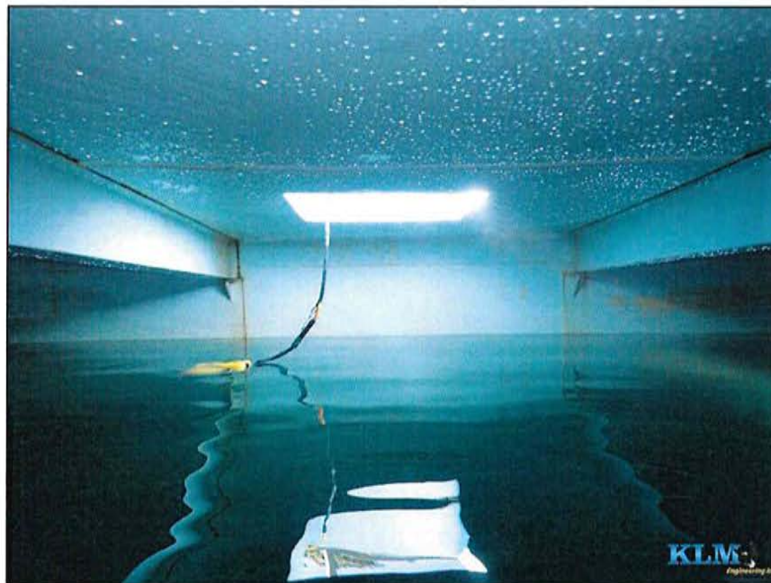
Photo No. 6 Condition of shell Wet access manway visible
