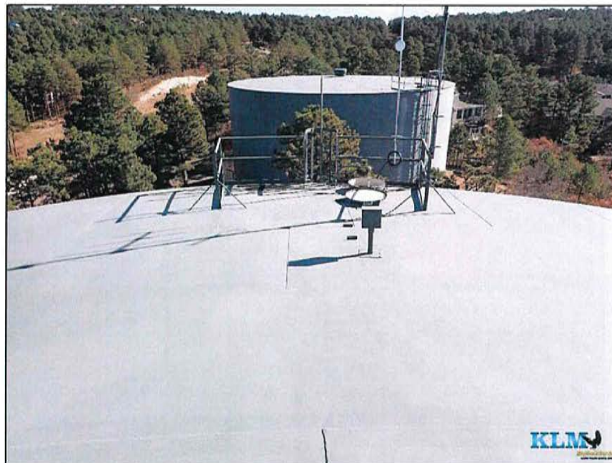
Photo No. 18 View of roof handrail and wet access manway
