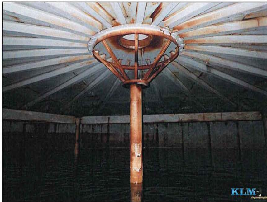
Photo No. 2 View of roof and center support column
