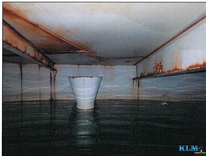
Photo No. 10 Condition of shell Overflow pipe visible
