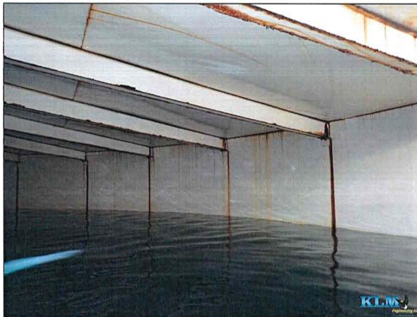
Photo No. 8 Condition of shell
