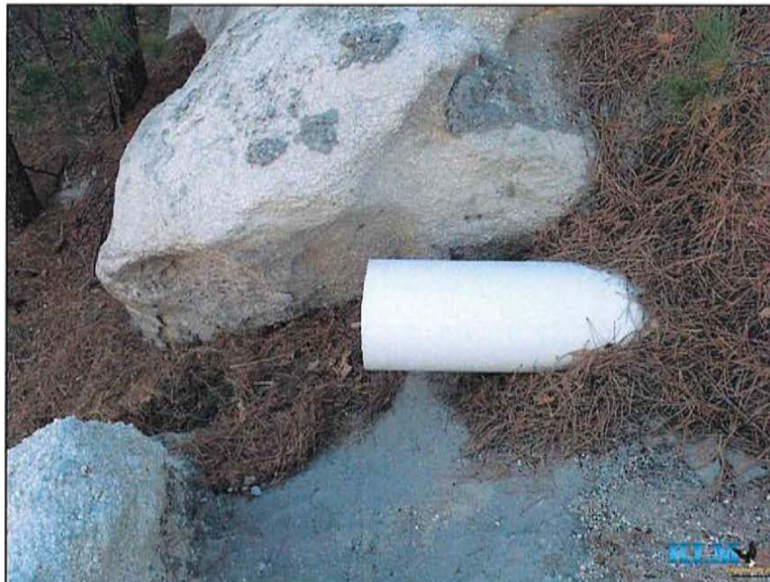
Photo No. 26 Overflow pipe outlet
