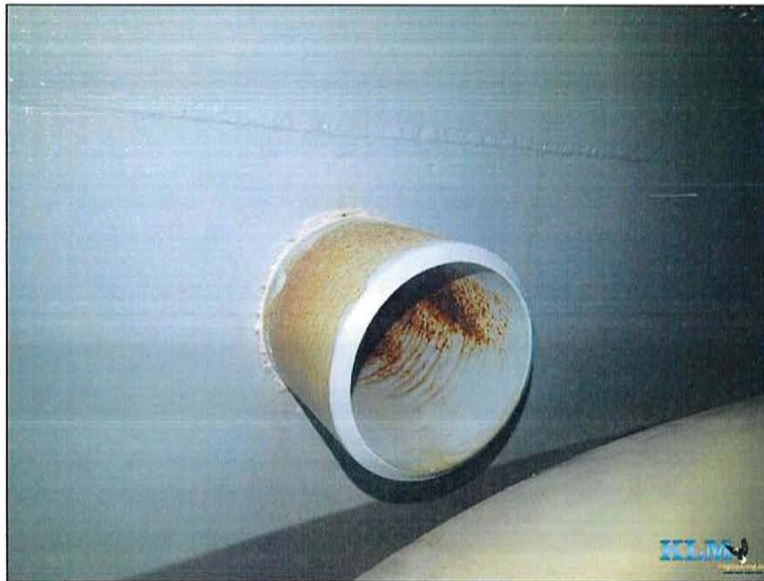
Photo No. 8 Condition of overflow pipe
