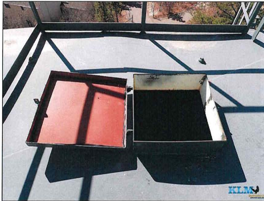
Photo No. 17 Condition of wet access manway
