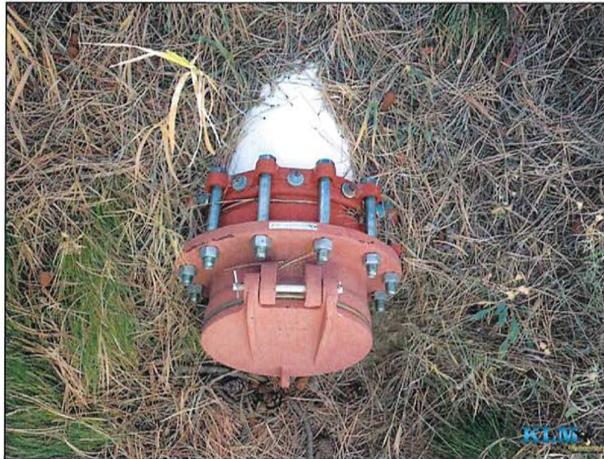
Photo No. 21 Overflow pipe outlet
