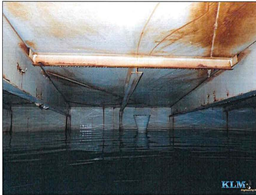
Photo No. 7 Condition of roof rafters and roof plates
