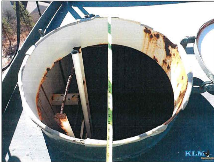
Photo No. 19 Condition of wet access manway
