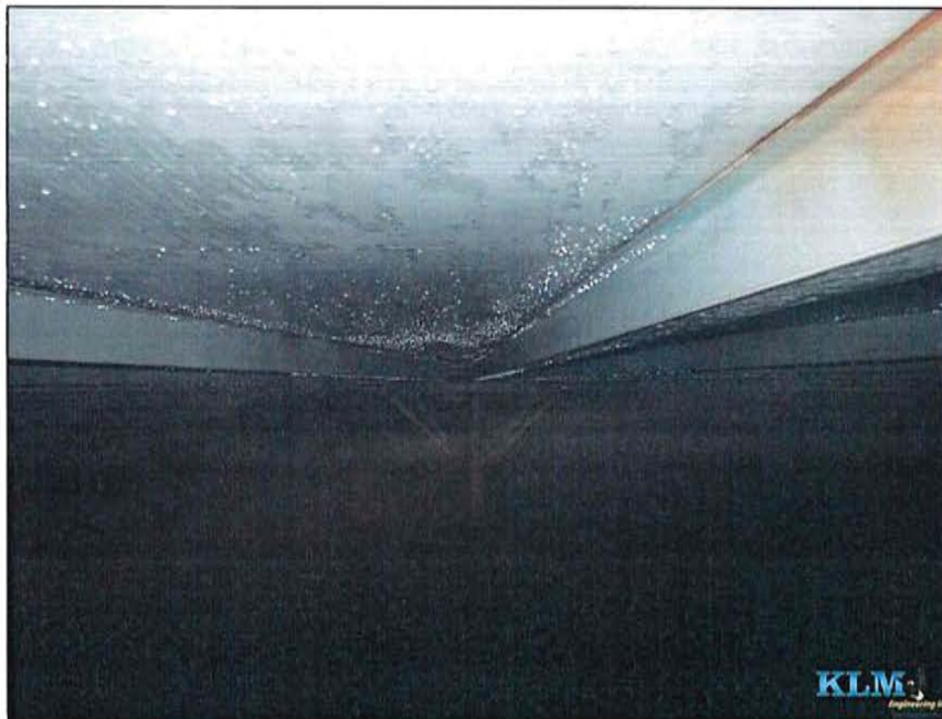
Photo No. 4 Condition of roof rafters and roof plates
