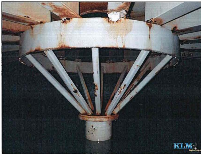
Photo No. 4 Condition of center support column
