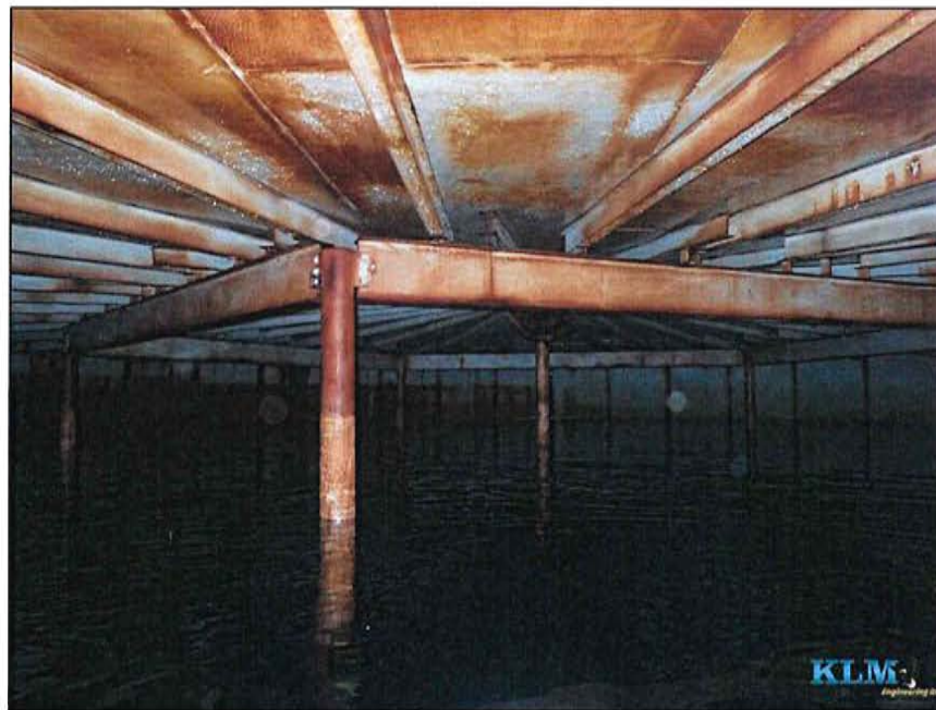
Photo No. 6 View of roof plates, roof rafters, and support columns
