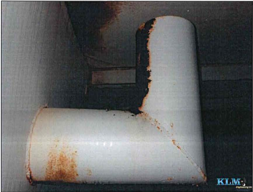
Photo No. 11 Condition of overflow pipe
