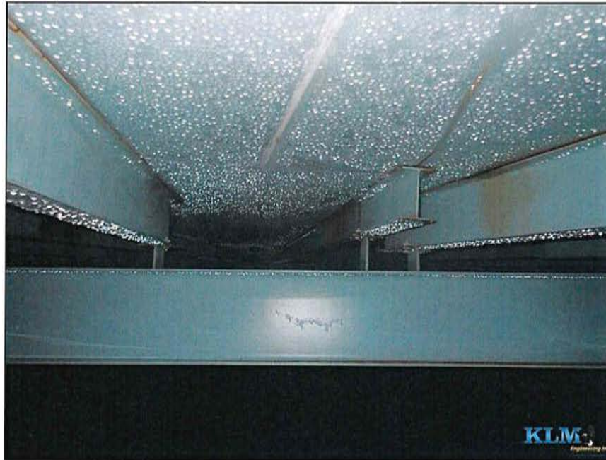
Photo No. 5 Condition of roof rafters
