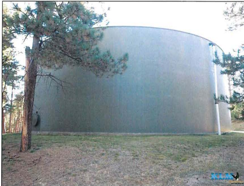
Photo No. 1 Overall view of reservoir
