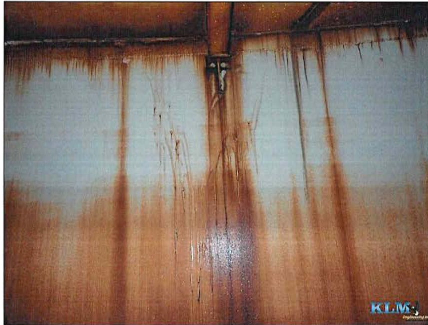
Photo No. 11 Condition of shell
